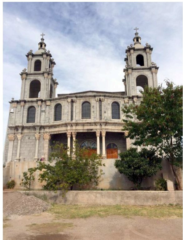
The enigmatic Iglesia de la Virgen de Fatima in Magdalena, Sonora. Built by two brothers who had a vision, or calling. Construction began ~1980 and the church is still not fully finished, although it is functional. In front are two "Kino Heritage Fruit Trees," a peach and a loquat (and a large el Guaje tree on the right, from far to the south).
