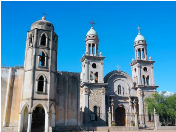
The town and mission at Baviácora, Sonora, were founded by the Jesuit Bartolomé Castañón in 1639. The original church stands to the left of the newer church, built by Franciscans in the 18 th century—Iglesia Nuestra Señora de la Concepción de Banácora.
