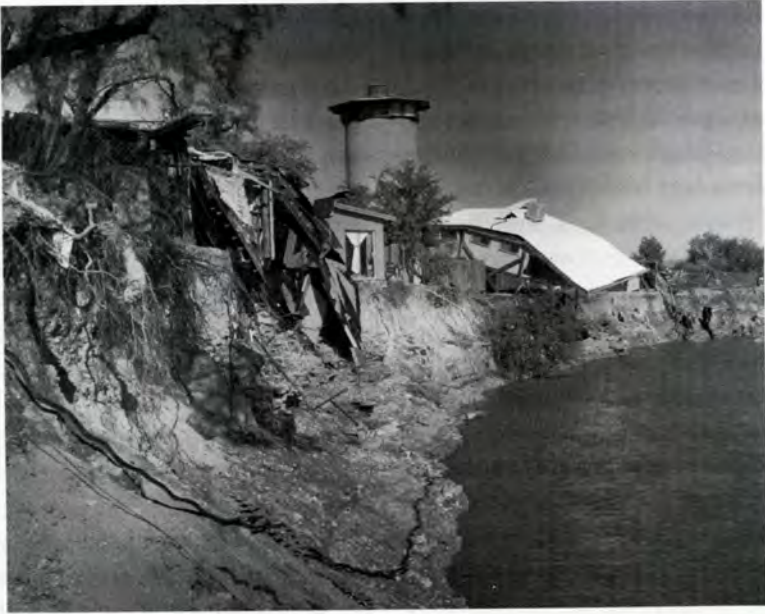
Flood damage along Tucson's Rillito River, October 1983
