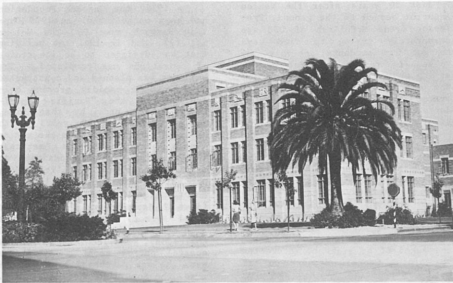
Fig. 4. The Allan Hancock Foundation. circa 1943.
